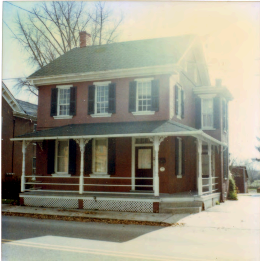
20 East Main Street, prior to restoration
