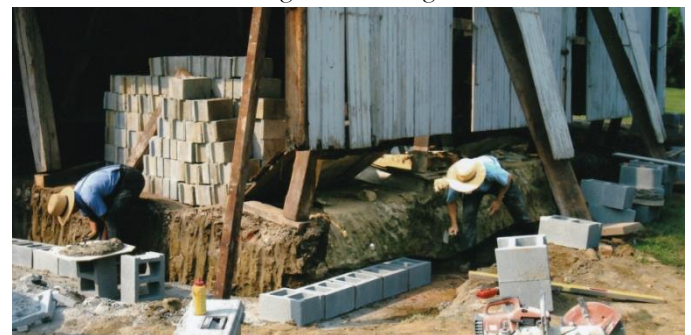
above: The barn, prior to restoration below: "barn raising" – rebuilding the foundation
