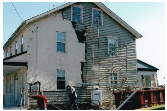
above: 313 Miller St. house, prior to restoration work below: Peeling away the stucco on the west side of the house
