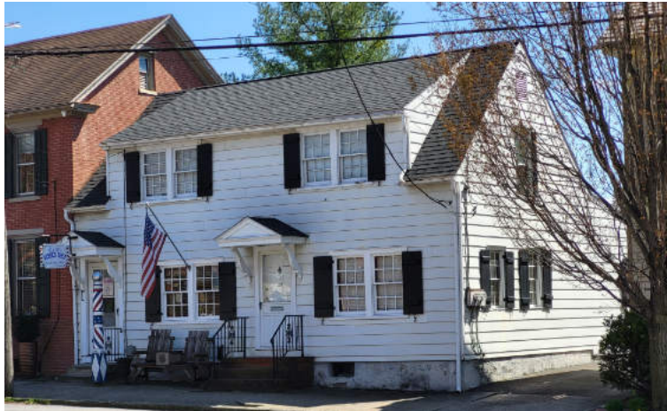
The white siding on the house at 20 West Main Street conceals the original log structure built in William and Abigail Phillips circa 1751.
